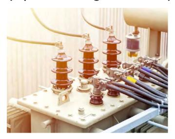
A phase-shifting transformer is a device for controlling the power flow through specific lines in a complex power transmission network. The basic function of a phase-shifting transformer is to change the effective phase displacement between the input voltage and the output voltage of a transmission line, thus controlling the amount of active power that can flow in the line.
